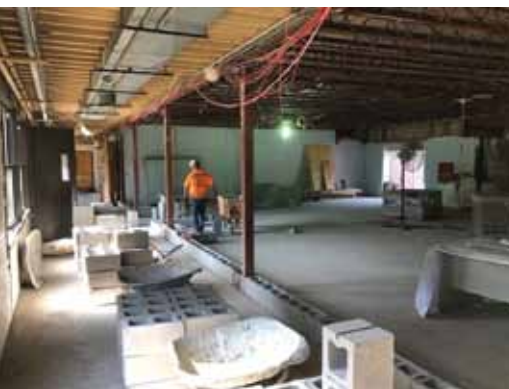
Renovations to the high school cafeteria and kitchen are in progress.
